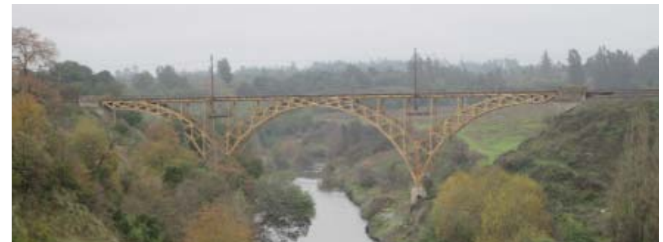
Rio Claro bridge
