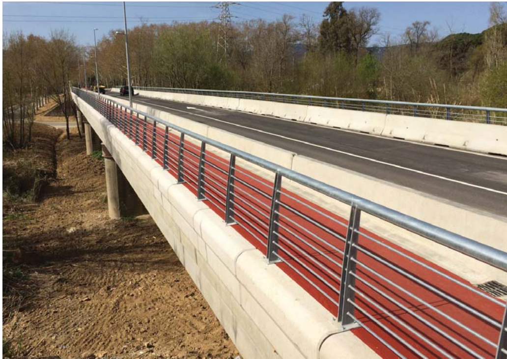
Railing on bridge 2.
