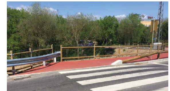
Single timber-steel guardrail.
