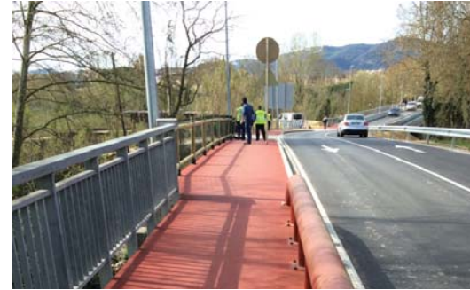
Tubular guardrail on Adif Bridge.
