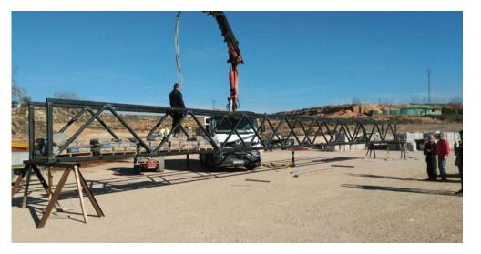
with two stair flights, which structure is based on two 250x100 mm tubular beams connected with crossbars, whereas the central module spans 25.00 m and it is designed as a Warren lattice type, 1.35 m thick.
