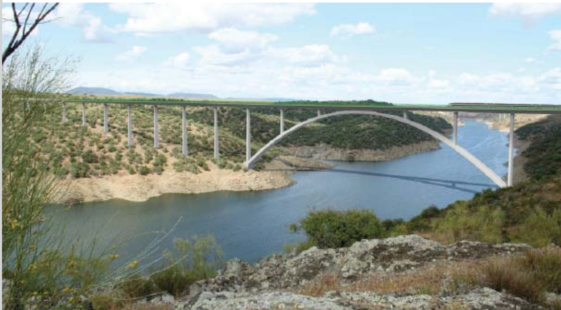
Construction process Construction process Construction process Construction
